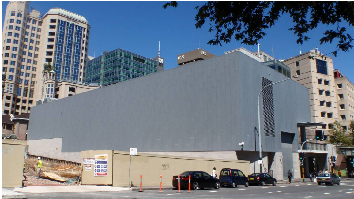
Figure 2: View of the substation from the north east on Ultimo Road.
