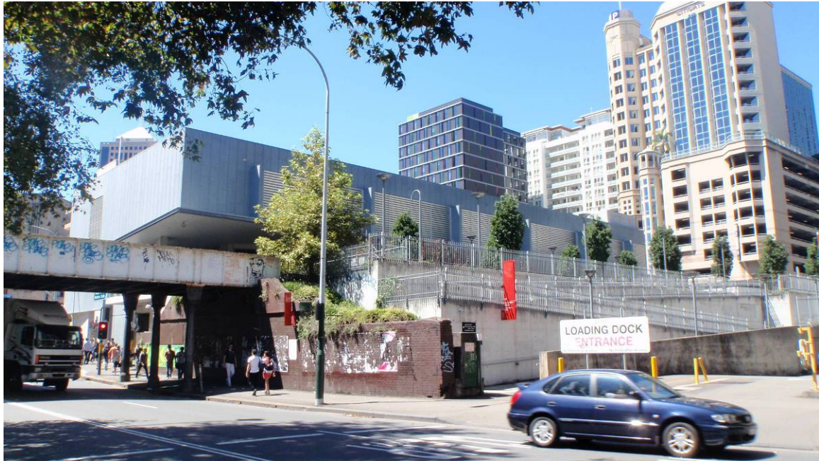
Figure 4: View of the substation from the north west, with access to the UPN in the foreground.
